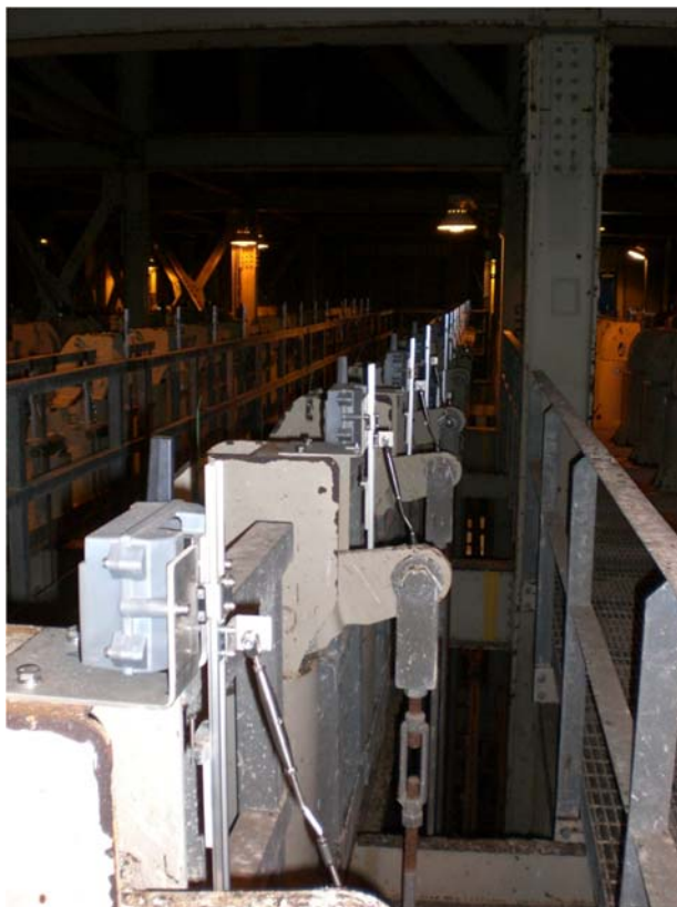
Figure 6: Real TGM field set up in a top fired reformer.
