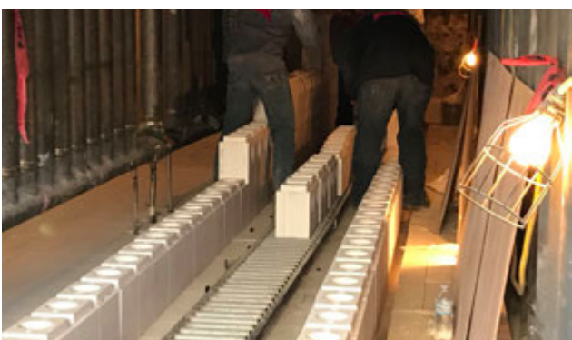
Figure 5. Building the walls.
