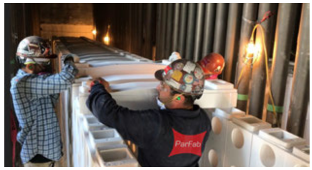
Figure 8. Installation of the lids.
