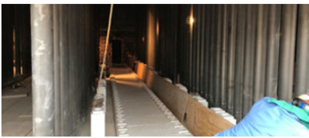
Figure 4. Base blocks complete.
