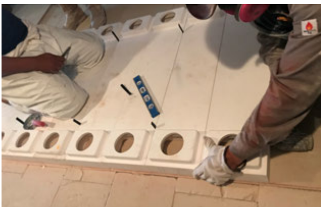
Figure 3. Placement of base blocks.
