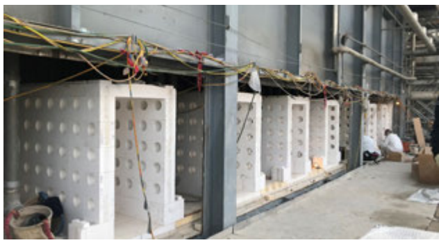
Figure 11. Nine tunnels constructed in one week.
