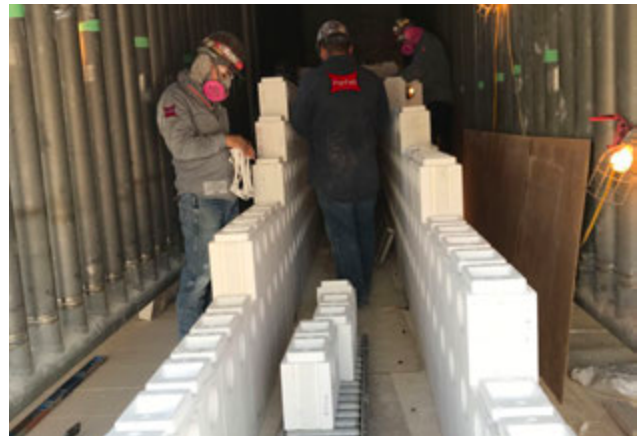
Figure 6. Placing ceramic fiber gaskets between layers of blocks.
