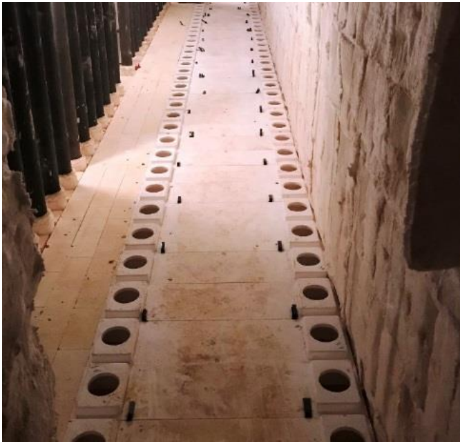
Figure 1. Tunnel Base Plates Installed
