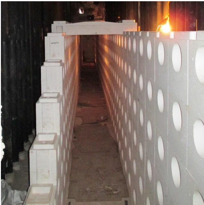
Figure 2. Partially Assembled Tunnel
